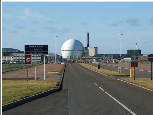
The Dounreay Nuclear Power Research Establishment as it was in 2006
